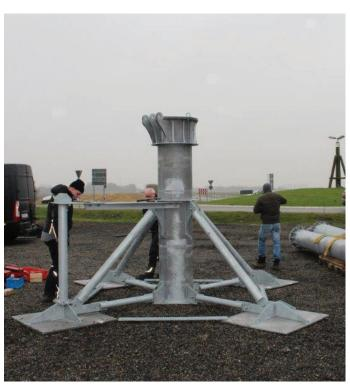
once the telecommunications technicians had mounted the antennae. This is an enormous time-saving in comparison to conventional concrete foundations", reports the ingenious entrepreneur. Naturally, he had to submit all statics, planning and safety verifications anchored in construction legislation for the erection of the mast.
