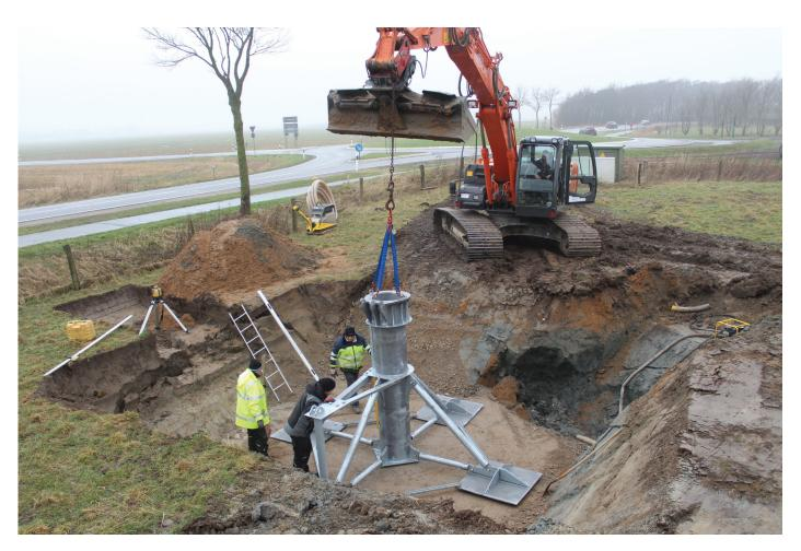
Whenever masts or towers have to be constructed, professional foundations are required. Foundations made from concrete are generally the most popular choice. Until now... the company BFtec from Nentershausen in Hessen wants to revolutionise the market with its so-called SteelRoots®. Company founder, owner and developer Peter Kellner is convinced that his steel root foundations without concrete will replace conventional construction methods in the foreseeable future.
