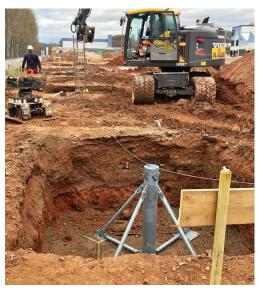
of the steel root foundations. Using a laser, the position height of the plates aligned are to the millimein order tre adhere to the accuracies and tolerances demanded in steel hall construction. They are then fixed using a few litres of concrete, for which the curing time is
