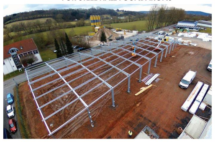
The first commercial hall in the world to be erected on steel root foundations without concrete now stands in the Haunecker district of Unterhaun in the administrative district of Hersfeld-Rotenburg. The Hersfeld-based construction company Räuber erected the building on the basis of SteelRoots® by BFtec, a company from Nentershausen-Süß.
