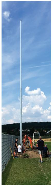
ground. Depending on the use and height of the mast, steel struts and plates are inserted into an excavation pit in a similar manner to the root system of a tree before being backfilled with the soil previously removed. This is far quicker to execute and involves less effort and expense than conventional concrete foundations. No formwork has to be provided, the concrete does not need to cure and no excess soil has to be transported away. Also, no crane is required to set up the mast.
