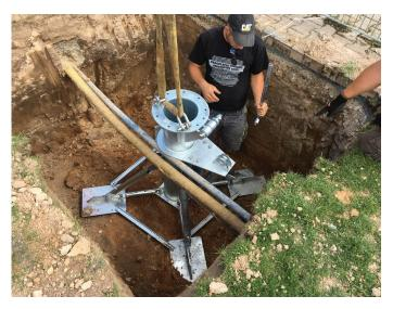
water supply pipes can be "incorporated" into this foundations system without the lines having to be capped. After this, the mast segments are plugged together and connected with the SteelRoots® via a folding joint.
